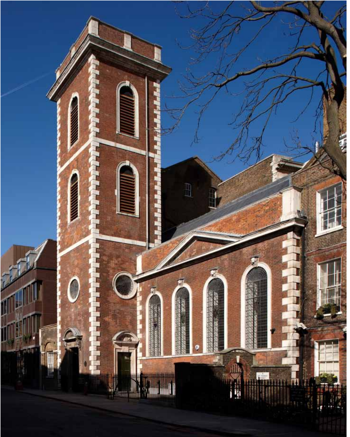
View from St Thomas Street
