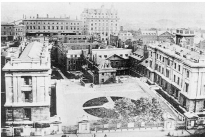
View of the modified courtyards from the late 1800's
